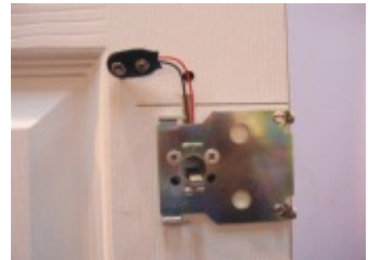
Step 7. Shows Rim Combi -with tails protruding through hole and battery wires aligned into the grooves.
