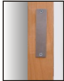
Step 1b. Battery pack mortised into side of door
