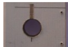
Step 4. Chiselling cut out for battery wires
