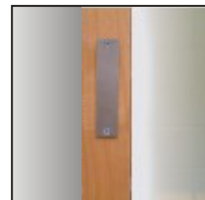
Edge of door showing mortice battery pack
