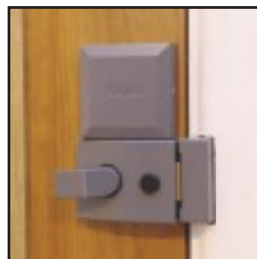
Inside of door - showing surface mounted battery pack
